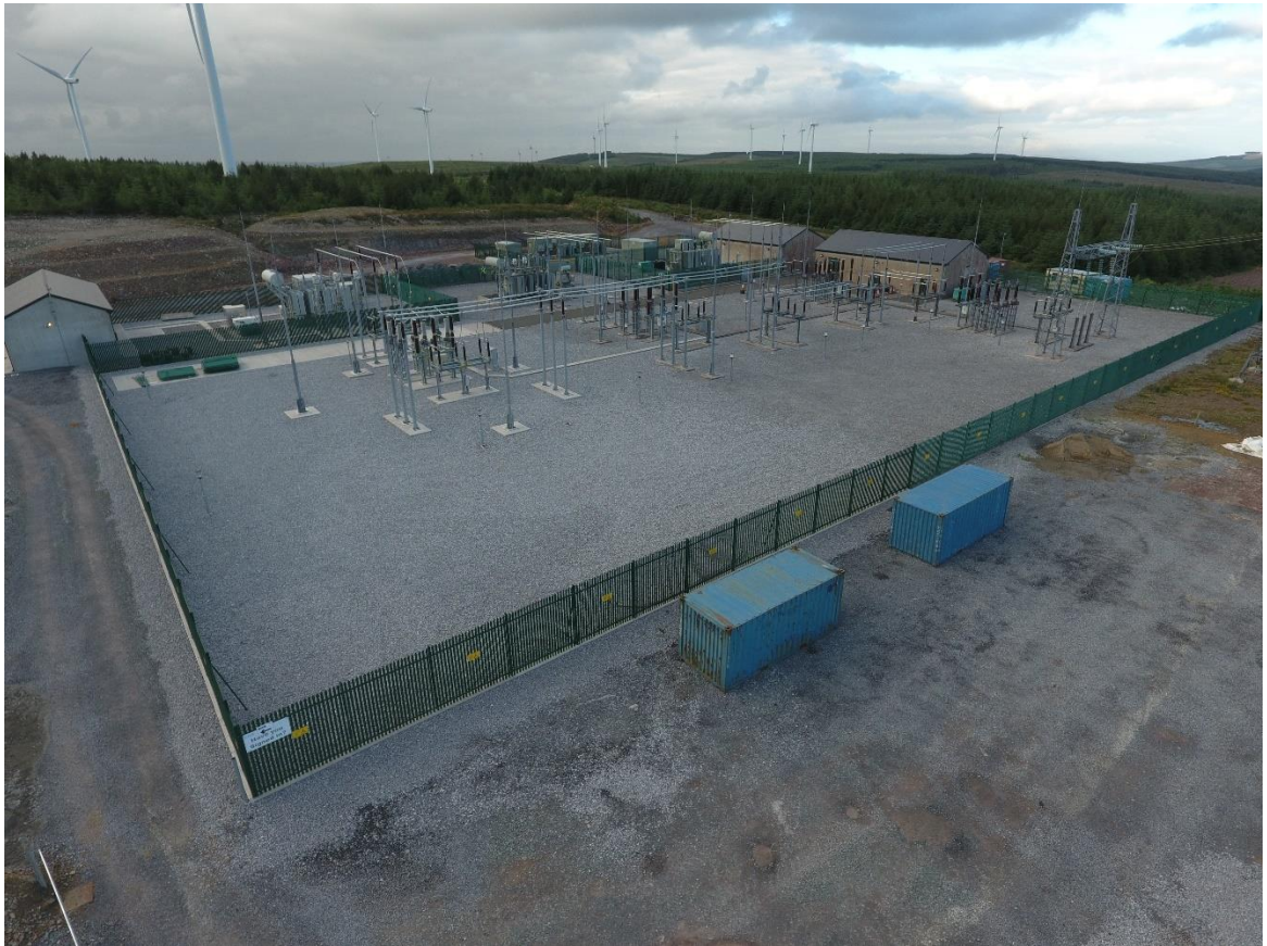
Photo 4.3 Typical 132kV substation compound
