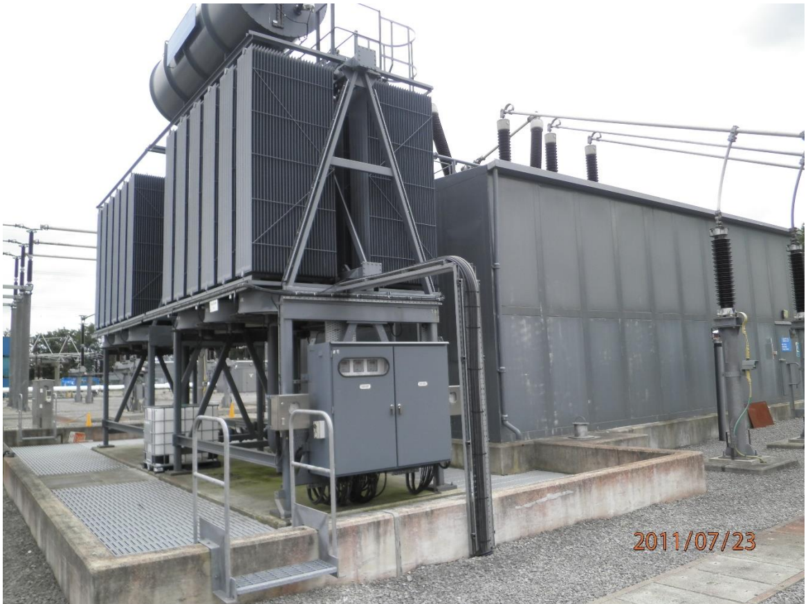
Photo 4.2 Typical (large 400kV) power transformer
